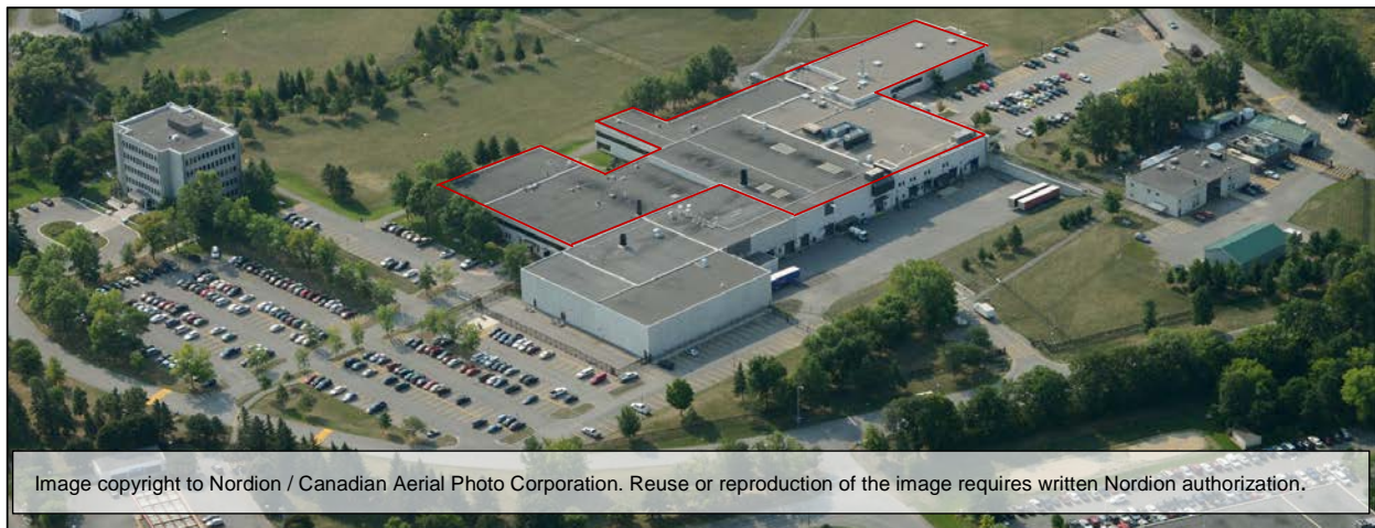
Figure 1: 447 March Road – Aerial View (BWXT Medical leased area outlined in red)
